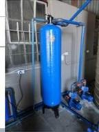
Typical Manual or Automatic MnO2 Iron Removal Unit & System in operation.
